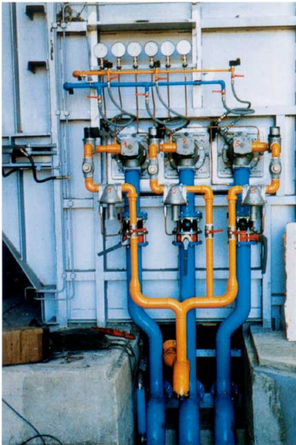
▲ Sequential burners, PLC controlled with charge initialisation
